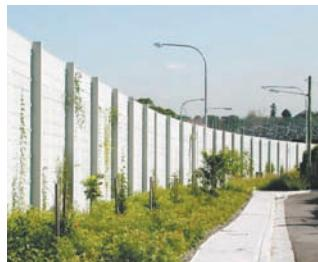
SoundBarrier panels are steel reinforced Hebel Autoclaved aerated concrete (AAC), a solid masonry product that is very strong yet 25% the weight of standard masonry and quick to install.
